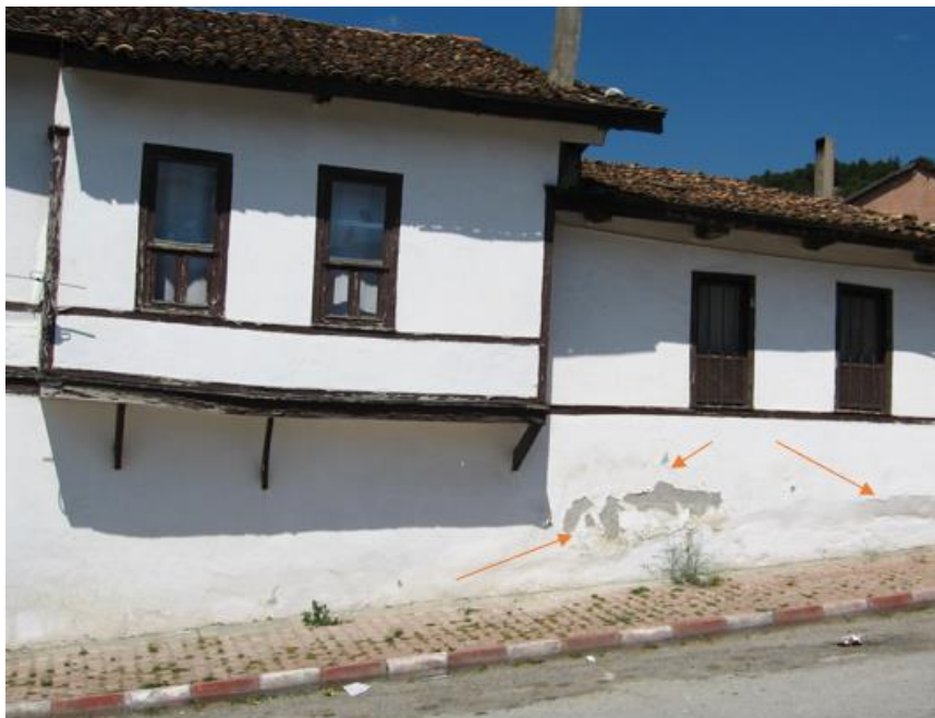
Figure 7. Nevzat Akay House of deteriorations caused by the effect of heat on the exterior of the sturcture.
